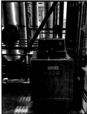
**IWD-12: Sampling port on the constantly recirculated slip stream at the F42 AWN-B train effluent and located on the ground level, discharging to the Water Treatment and Recovery facility (WATR), then to sanitary sewer.**
