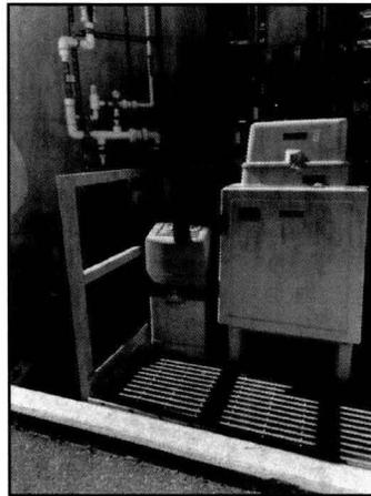
**IWD-2: Sampling port on 12" Discharge pipe following the third stage of the Fab 12 SLW treatment system and located along the ground level, discharging to the Water Treatment and Recovery facility (WATR), then to the sanitary sewer.**
