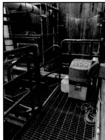
**IWD-8: Sampling port on 12" Discharge pipe following the third stage of the Fab 22 Awn treatment system and located along the mezzanine level, discharging to the Water Treatment and Recovery Facility (WATR), then to the sanitary sewer.**
